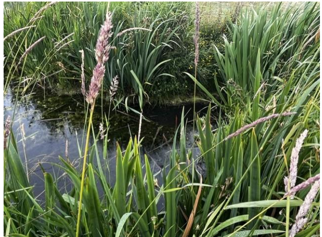
Far N.E. corner (near culvert): less plant debris present than last month. Duckweed nearly gone.
